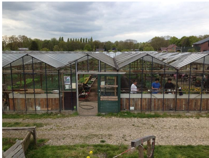
5. The greenhouse at the Koningshof
